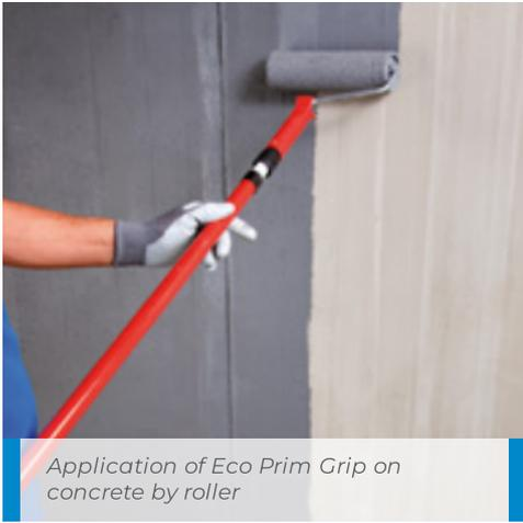
*Application of Eco Prim Grip on concrete by roller*
