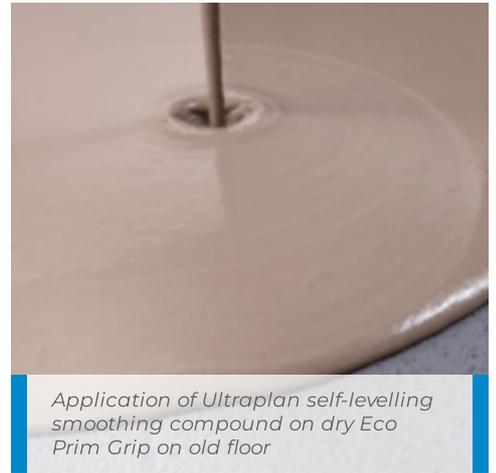
*Application of Ultraplan self-levelling smoothing compound on dry Eco Prim Grip on old floor*
